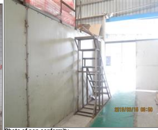
Photo of non-conformity stair without handrail and the platform higher than 2m used for packing materials storage lacked of guardrails in few areas.JPG
