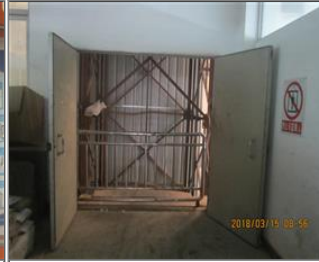
Photo of non-conformity safety door of easy lift without interlock.JPG
