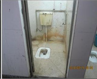
Photo of the sanitary facilities Toilet.JPG
